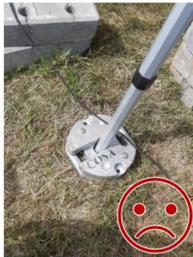
Figure 3. The counterweights are not interlocked. In this case, only gravity holds them together.
